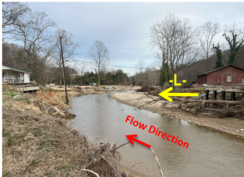
View of Bridge 740112 looking east
