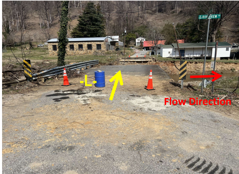
View at End Bent 1 looking north
